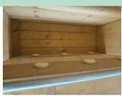
The owners of the shopping center decided that prevention was better than cure. So, in December 2015 approximately 9,000 dishes of Optical Gel were fixed to all the sheltered parts of the structure. (The covers were subsequently removed from the dishes.)
