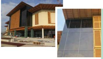
Even before construction was completed pigeons started to roost in sheltered parts of the building. Pigeons roosting below the roof were creating an unsightly mess on the glass façades
