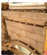
At the second floor, all nests were removed from below the curved lintel above the central window, from below the inverted V-shaped lintels on either side and from the architectural features to left and right. All these surfaces were treated with dishes of Optical Gel at 6 in centers to prevent nesting.
