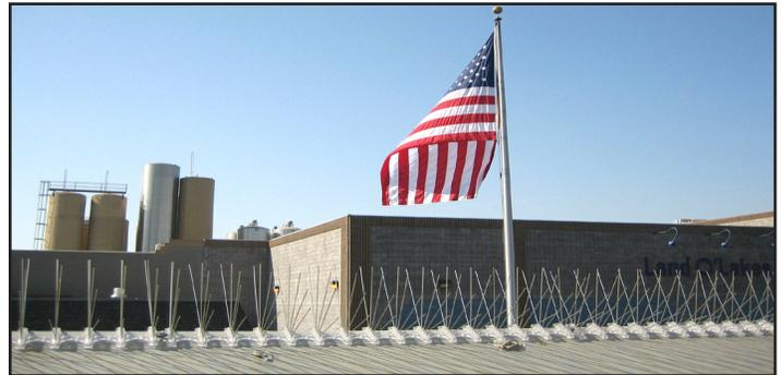
MasterLine™ Stainless Steel Bird Spikes installed on a parapet wall.
