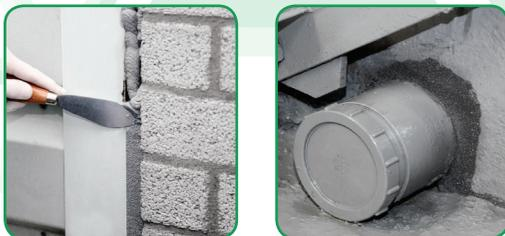
RodentStop is an effective product to seal seams, cracks and holes to prevent entry from rodents and other pests.
