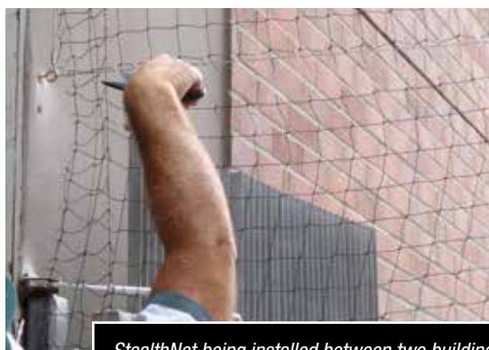
StealthNet being installed between two buildings to keep pigeons away from sensitive equipment.
