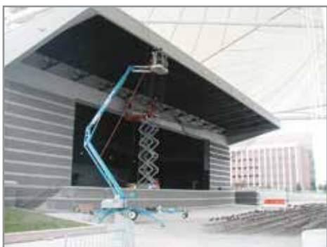
A Bird Barrier Certified Installer installs horizontal StealthNet under this theatre overhang to keep sparrows from perching on the beams and pipes over the stage.
