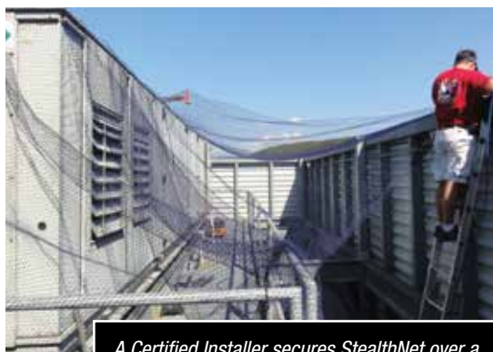
A Certified Installer secures StealthNet over a hospital's HVAC system to exclude birds.
