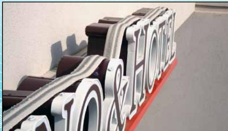
**Bird Jolt Flat Track is completely flexible conforming to any surface.**
