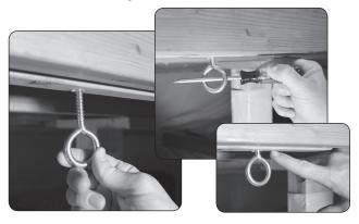
**Step 4:** Distance the second eye bolt 35" away from the first eye bolt on the same joist and screw into place.
