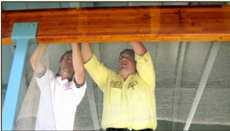
Bird-B-Gone manual hog ring tool makes bird netting installations a "breeze"!
