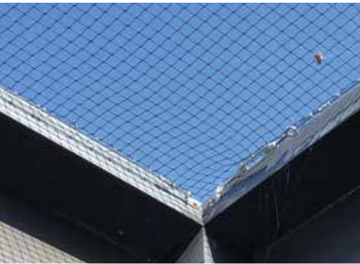
StealthNet secured to a large barrier around rooftop HVAC equipment.
