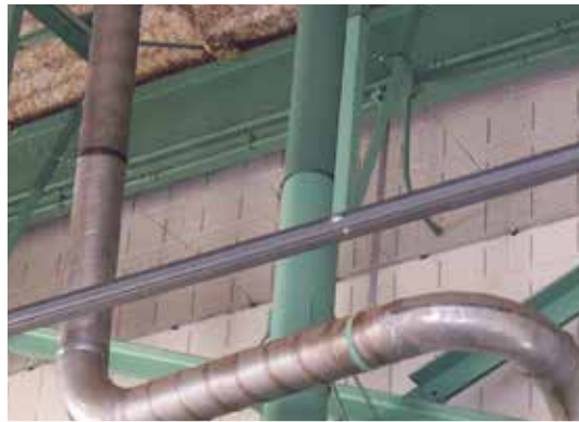
An intricate installation around pipes keeps birds from entering the protected space.
