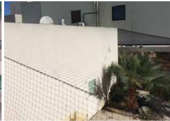
A hospital courtyard is protected from pigeons by 2" StealthNet suspended overhead.
